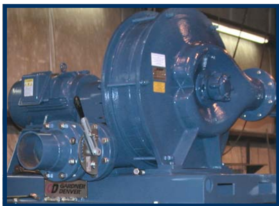
Gardner Denver 4203A exhauster and 20 HP motor on Vac-1000 filter
